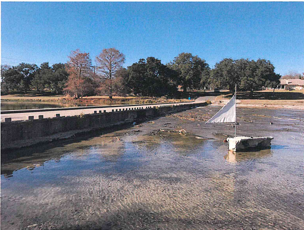
Figure 6 – View from East Side of Crossing Looking West
