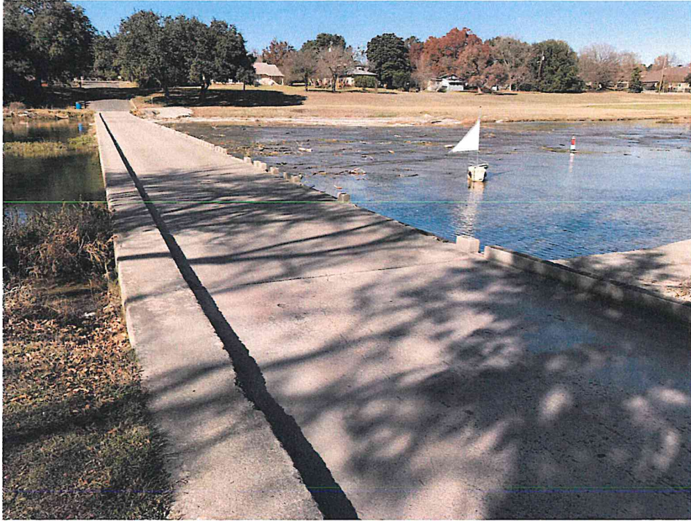
Figure 1 – View from Southeast End of Crossing
