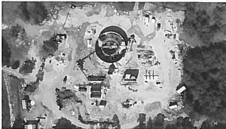
Figure 1 – Village of Salado Wastewater Treatment Plant
